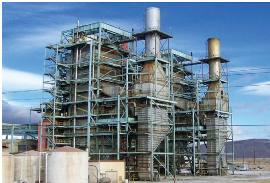
Fort Churchill Generating Station, in Nevada | NV Energy
