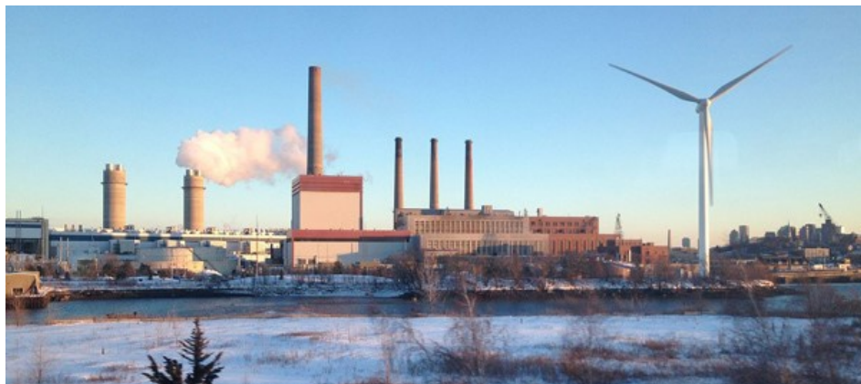
Mystic Generating Station
