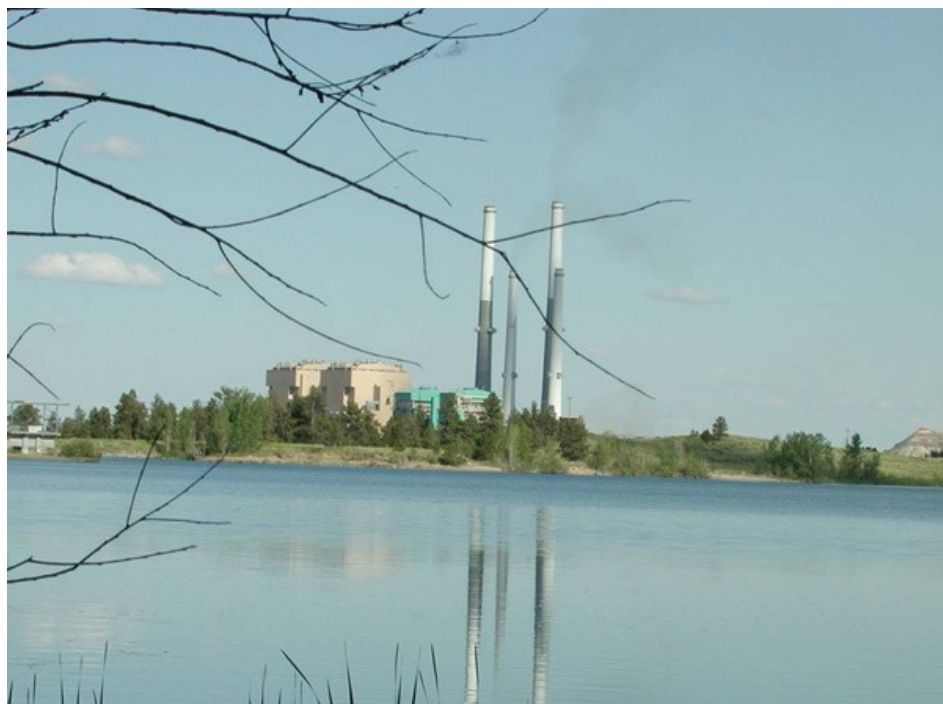
Colstrip Power Plant | Talen Energy
